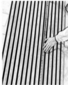
② Measure the wooden slat acoustic panel
