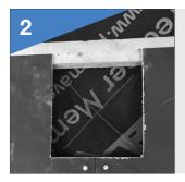
Mark a cut line 220mm x 60mm on the two slates below where the Vent is to be fitted, cut out the section and mark the underlay for opening into the roof space if required for future ventilation of connection to Flexipipe
