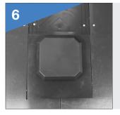
Continue by fixing the Slate Vent into the next course of Slates, fixing into the Tile Battens
