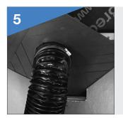
If the Slate Vent is just being used for roof ventilation fit the Slate Vent Adaptor ULTI3SVA and/or also with a Ulti-Mate Flexipipe ULTI3FP for connection to Soil Pipe of Mechanical Extraction, this will require the Underlay to be cut as shown in Section 2
