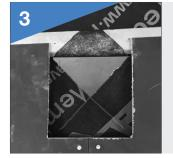
Fold back underlay with top section to the fixed to the batten above the opening.
