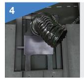
Select the Vent Tile to match to profile and colour and fit either without a flexipipe (if just being used for roof ventilation) or with a Ulti-Mate Flexipipe ULTI3FP for connection to Soil Pipe of Mechanical Extraction.
