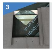
Cut the underlay as marked out and lift the cut sections with top section this is to the fixed to the batten above the opening.
